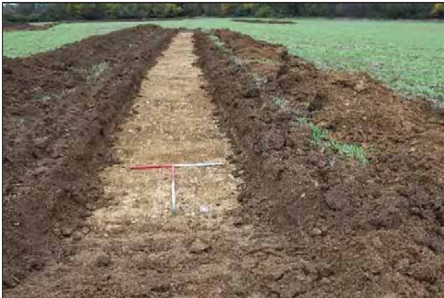
General view of Trench 6
