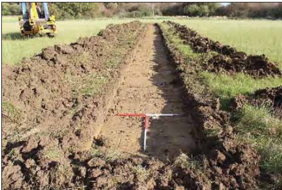
General view of Trench 30
