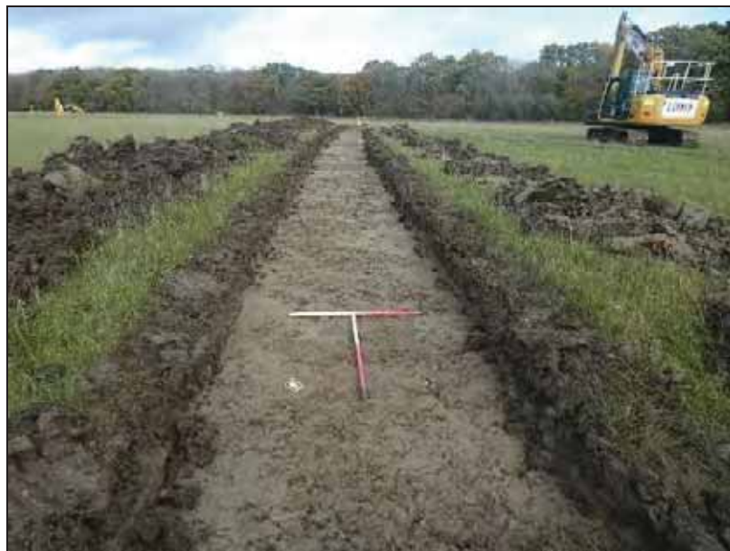
General view of Trench 24
