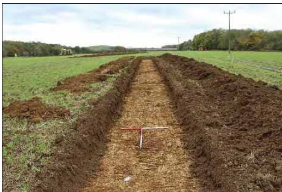
General view of Trench 4
