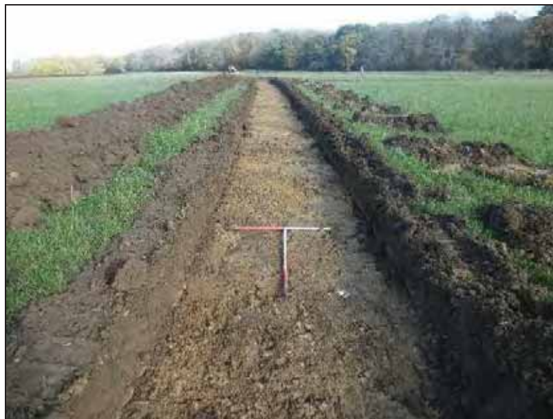
General view of Trench 18
