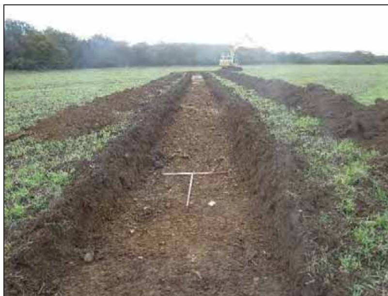
General view of Trench 13
