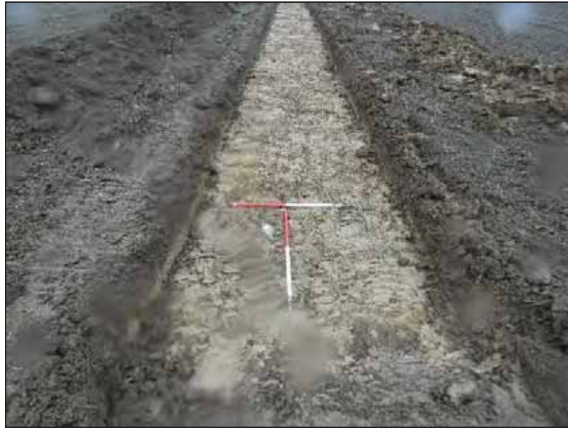
General view of Trench 44
